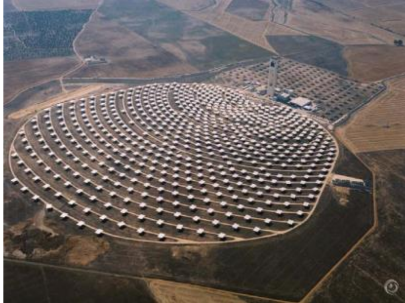
Figure 3: PS10 Solar Thermal Power Plant
