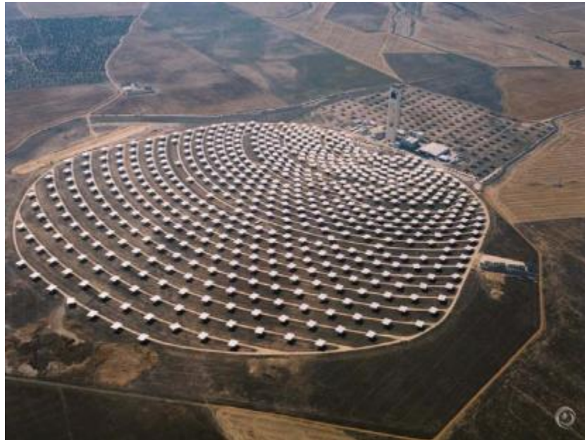
Figure 3: PS10 Solar Thermal Power Plant
